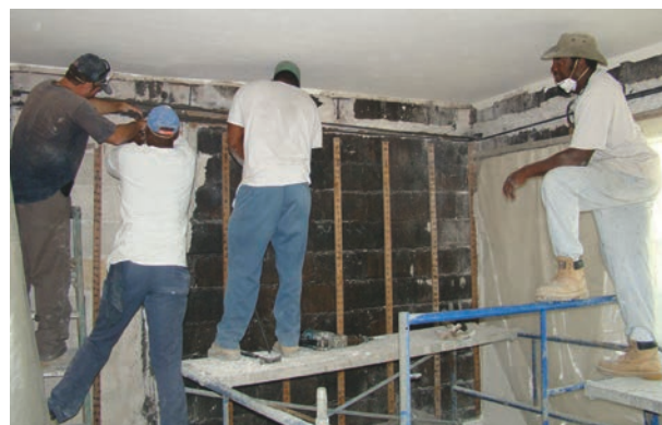
Concrete restoration of the Arthur Montgomery Guesthouse
