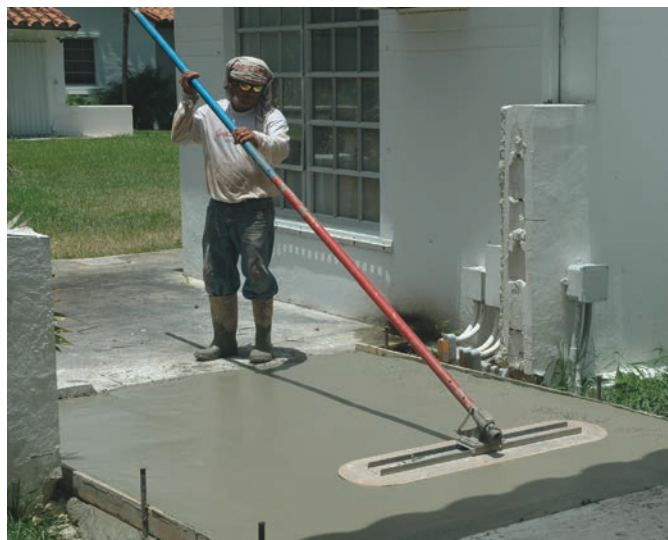
Concrete being smoothed at the Chris Tyson Plant Conservation Building
