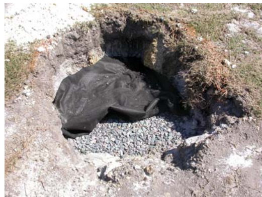
B. Gravel drainage layer (4") and filter fabric.
