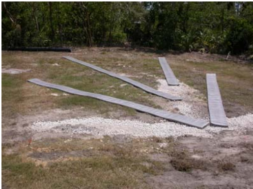
A. Dry well trenches and flat drainage pipe.
