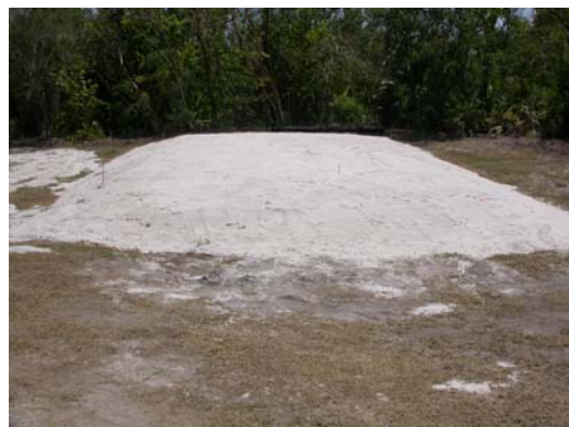
D. Coarse sand over filter fabric (18").
