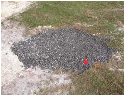
I. Completed pit with gravel mulch (3").
