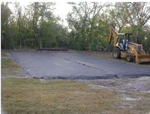
C. Filter fabric over drainage layer.
